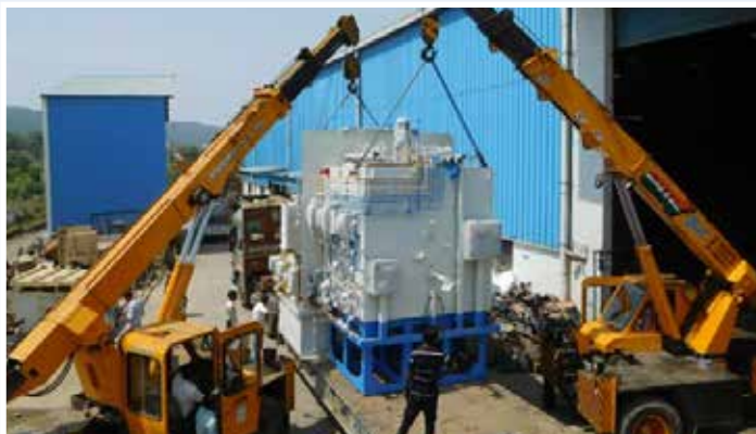
Loading of ODC's – Two cranes working in tandem
