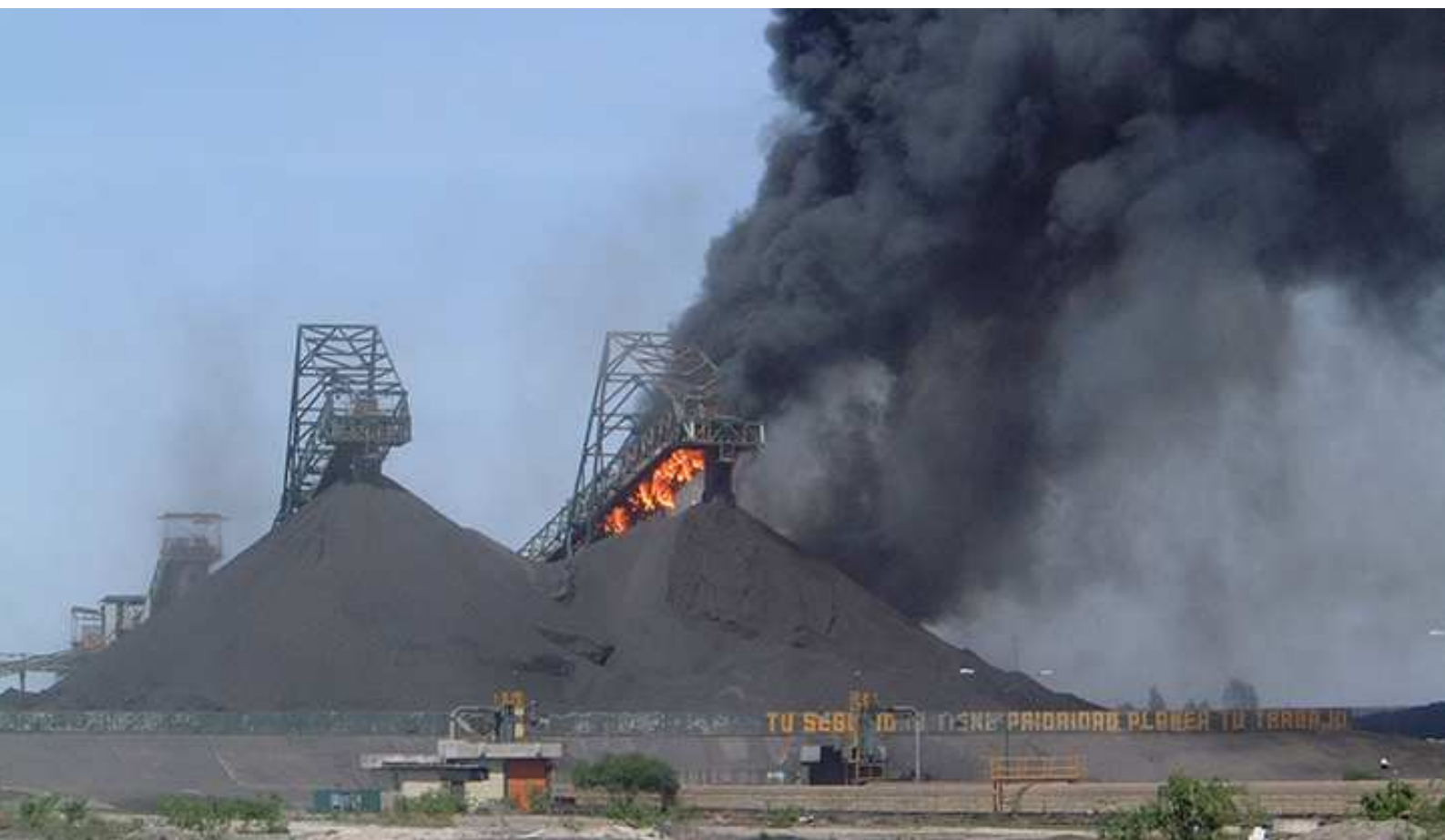
A rapidly spreading fire in a coal storage facility. Polymeric materials in the belt further worsen the situation
